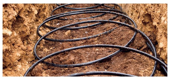
**Geothermal Coils:** Eight feet underground, this coil serves as part of a geothermal system enabled by Dow technology to heat and cool homes, schools and businesses.
